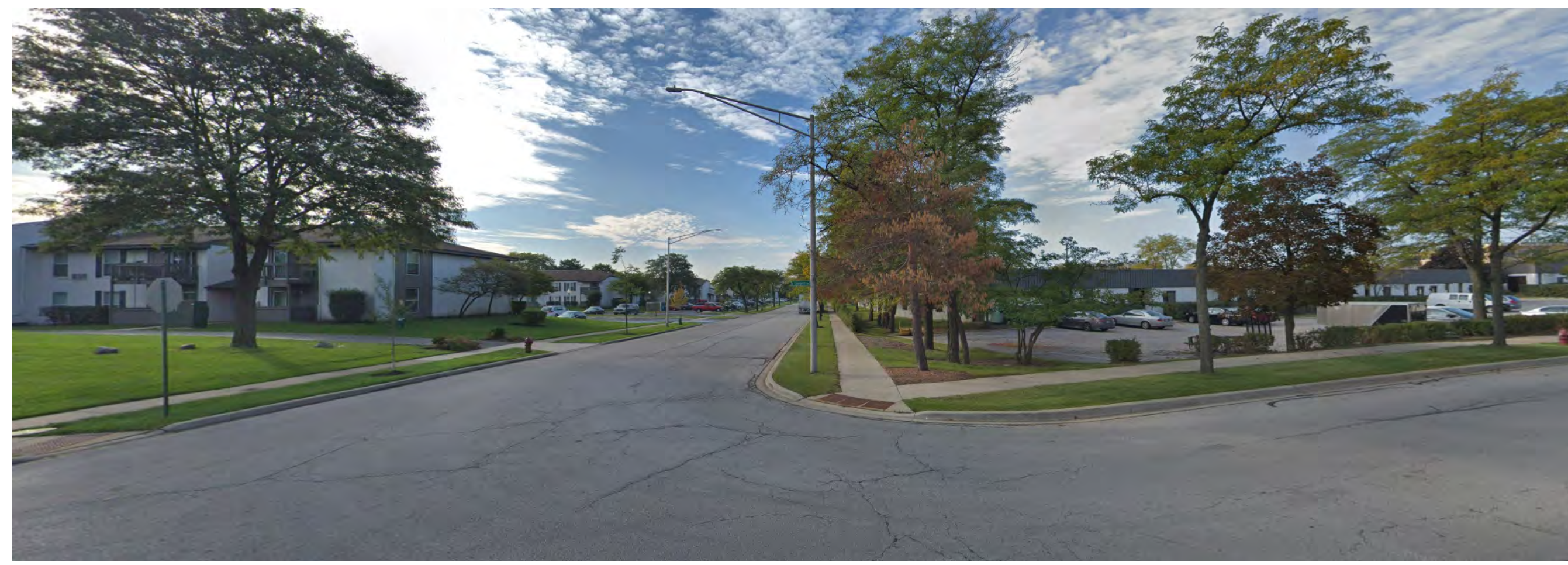
5 STREET VIEW - FROM NE CORNER, LOOKING SOUTH
