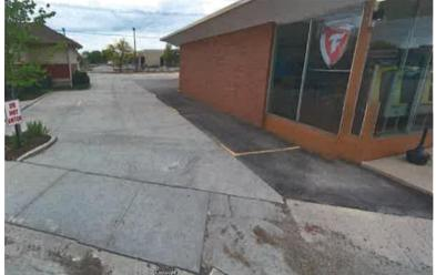
Note that the grading in this area has been adjusted so that the pavement elevation on our site matches the pavement elevation on the adjoining parcel. This will create a situation where the curb will be raised and act as a barrier between the two properties. There is no longer a danger of someone not realizing there is an elevation difference and driving over the curb.
