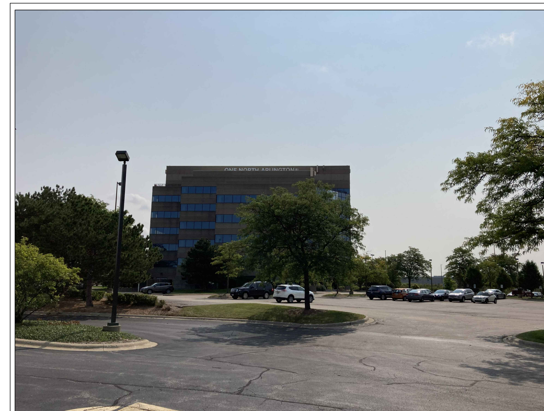
PROPERTY TO THE SOUTH
