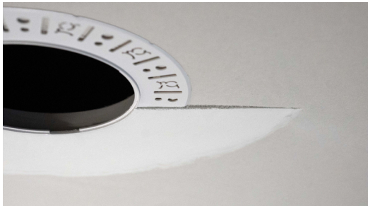
Partially finished mud ring, showing cross-section detail.
