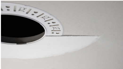
Partially finished mud ring, showing cross-section detail.
