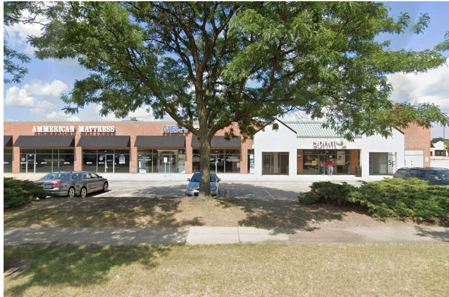
PROPERTIES WEST OF PROJECT SITE VACANT - PREVIOUSLY SPRINT STORE - 720 E. RAND ROAD NEXT DOOR & WINDOW - 718 E. RAND ROAD AMERICAN MATTRESS - 712-714 E. RAND ROAD
