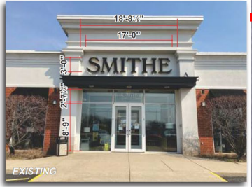
Southwest Elevation - Sign#6 - Before Existing Square Footage 46.5
