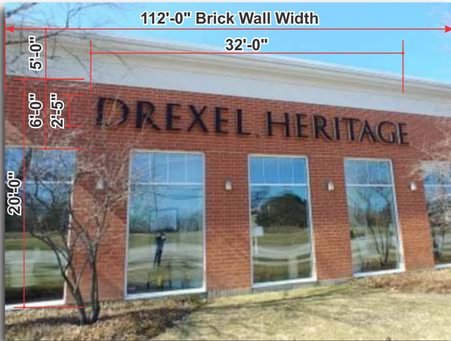
Northeast Elevation - Sign#3 - Before
