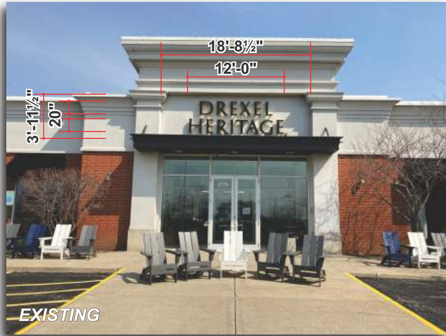
Southwest Elevation - Sign#1 - Before
