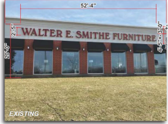
Northwest Elevation - Sign#4 - Before Existing Square Footage 126.5
