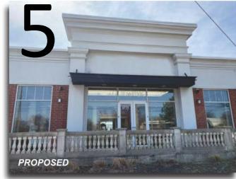
Northwest Elevation - Sign#5 - AFTER
