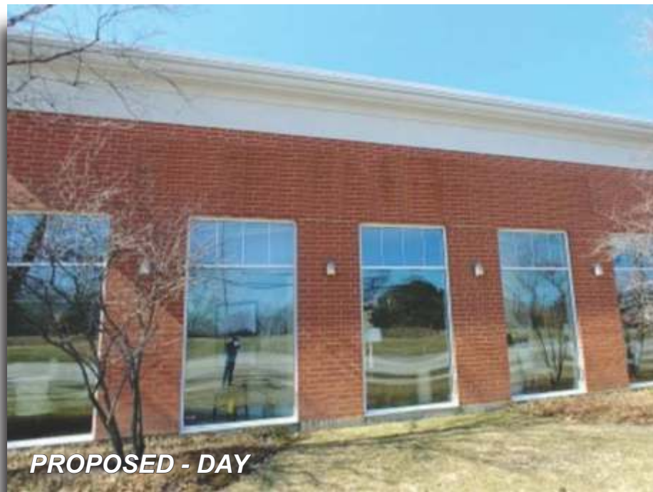
Northeast Elevation - Sign#3 - AFTER
