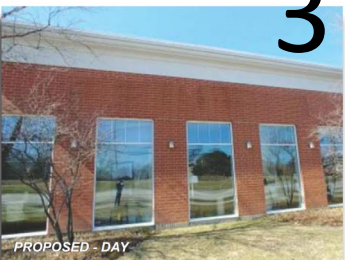
Northeast Elevation - Sign#3 - AFTER
