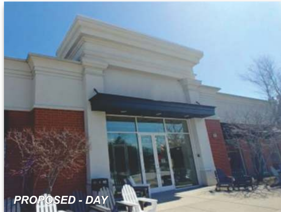
Southwest Elevation - Sign#1 - AFTER
