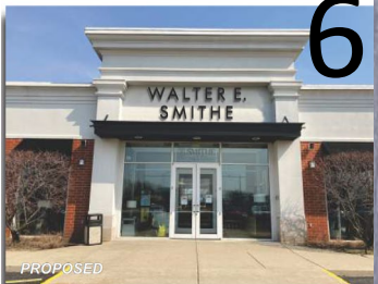
Southwest Elevation - Sign#6 - AFTER
