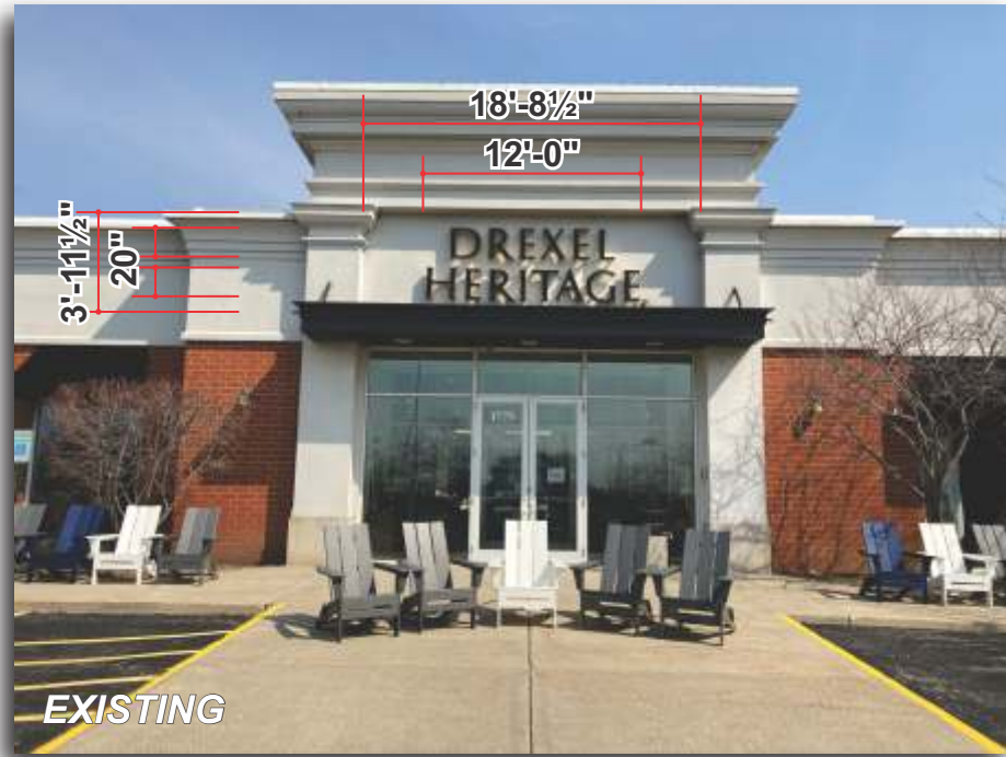
Southwest Elevation - Sign#1 - Before
