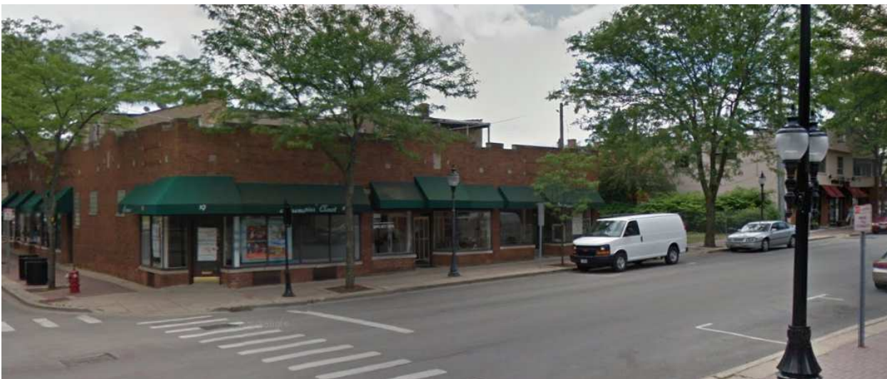
Image 2. View of vacant site from the intersection of Miner Street and Evergreen Avenue.
