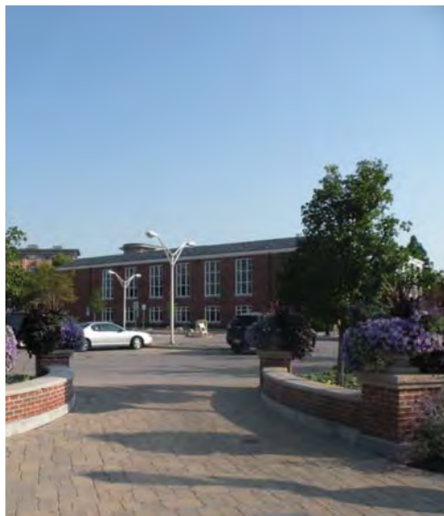
Garden walls at pedestrian access into parking lot
