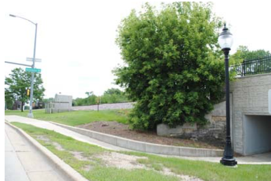
Northwest Highway (near the Davis Street underpass)
