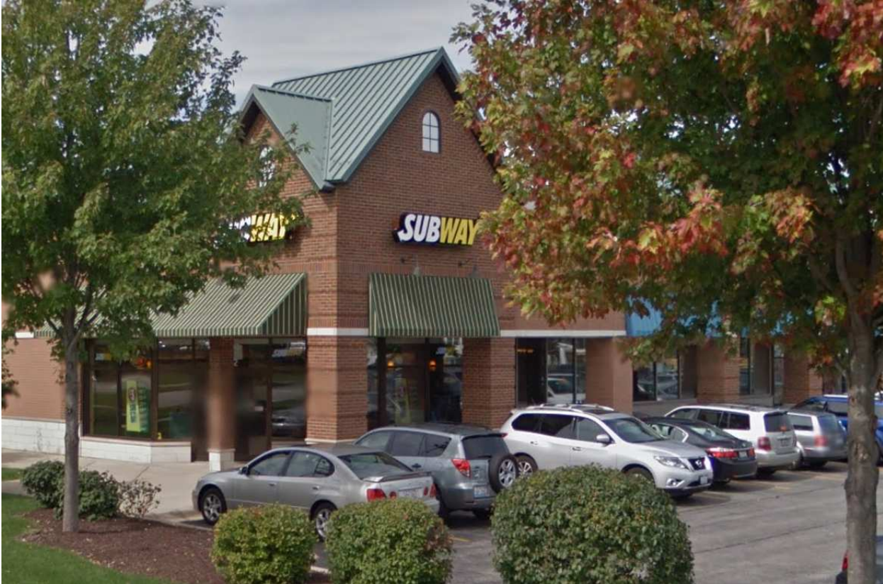
Image 1. Existing multi-tenant retail building as viewed from Kensington Road.
