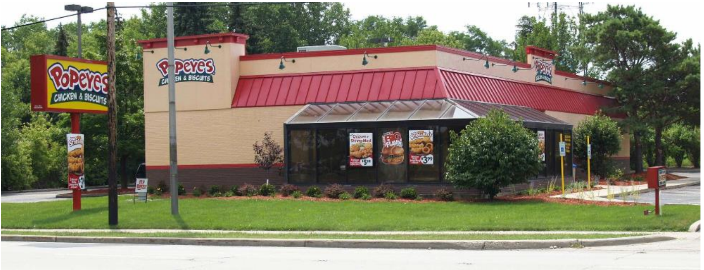
Photo 1. BEFORE PHOTO. Popeyes Restaurant and signage before the renovation.
